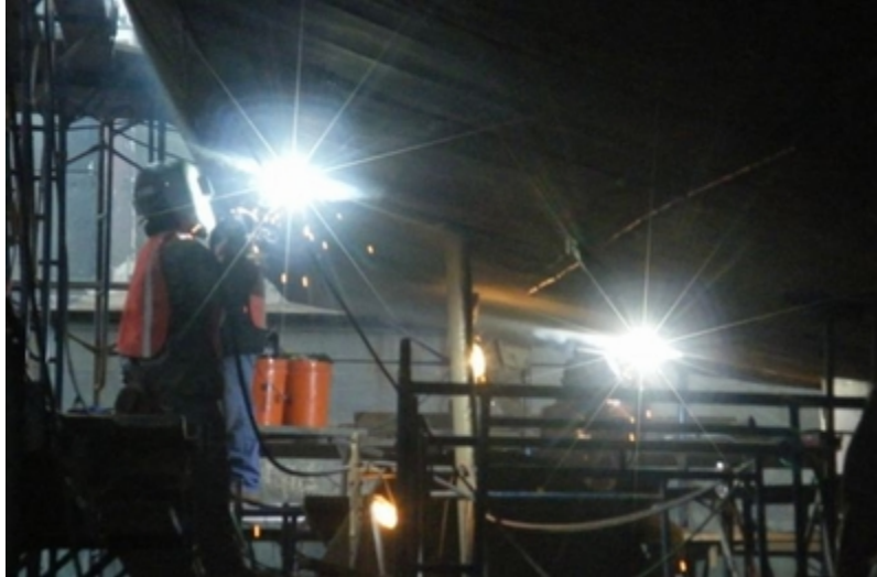
Welders installing new shell plating under the counter, U.S.S. CASSIN YOUNG.
