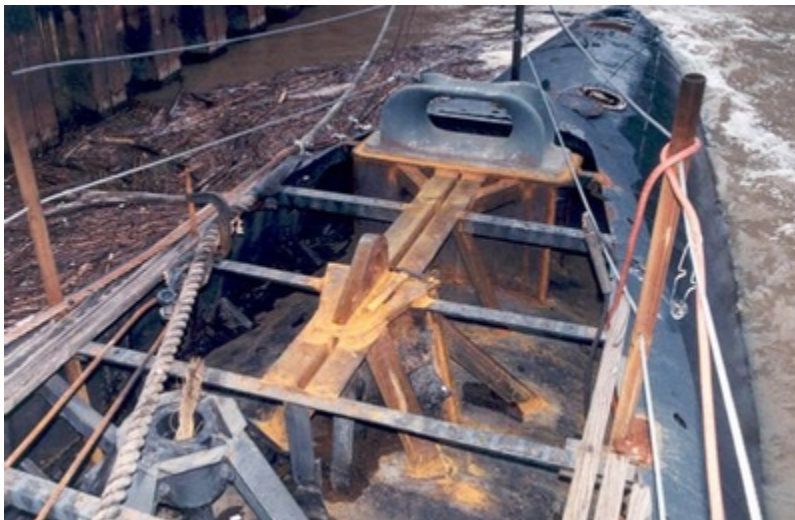
Installation of towing eye, stern chock and support structure to submarine U.S.S. CROAKER (SSK-246).
