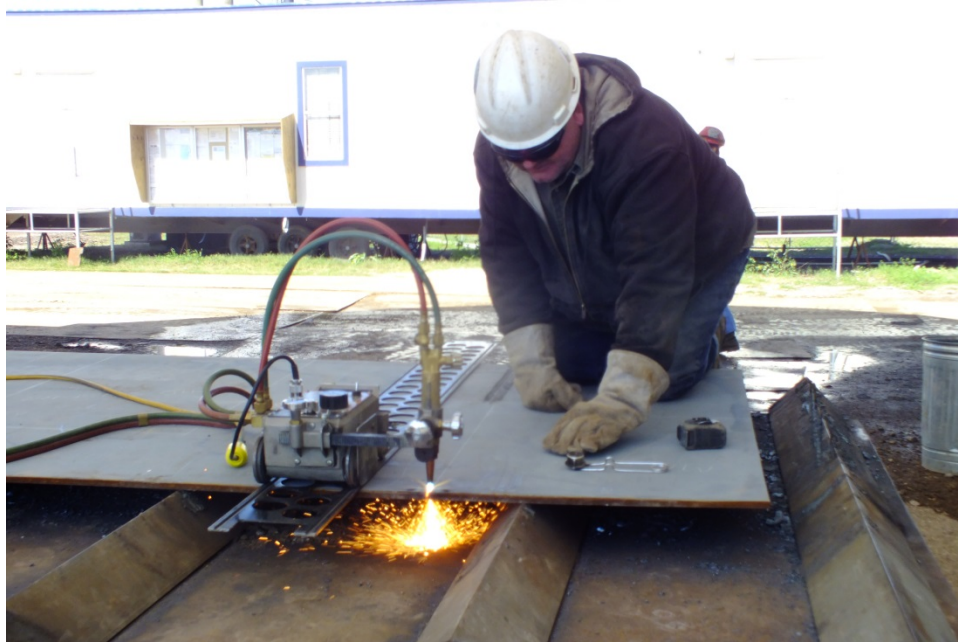
Track cutting of 3/8" plating for new framing aboard battleship U.S.S. TEXAS.
