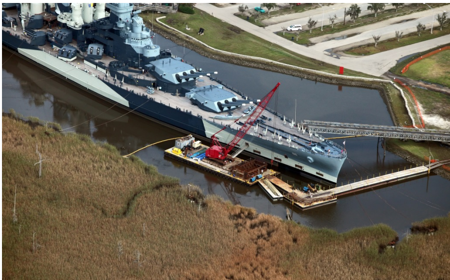
Aerial view of starboard bow of battleship U.S.S. NORTH CAROLINA, showing mobilized repairs underway.
