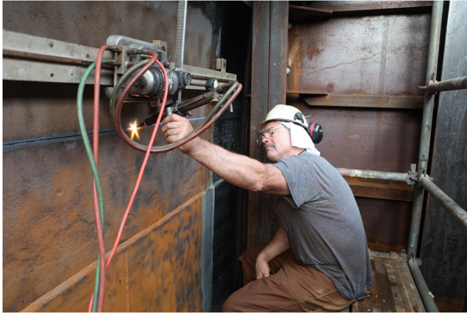
John Walker monitoring plasma cutter within portable cofferdam alongside hull, cutting away deteriorated underwater plating of battleship U.S.S. NORTH CAROLINA.
